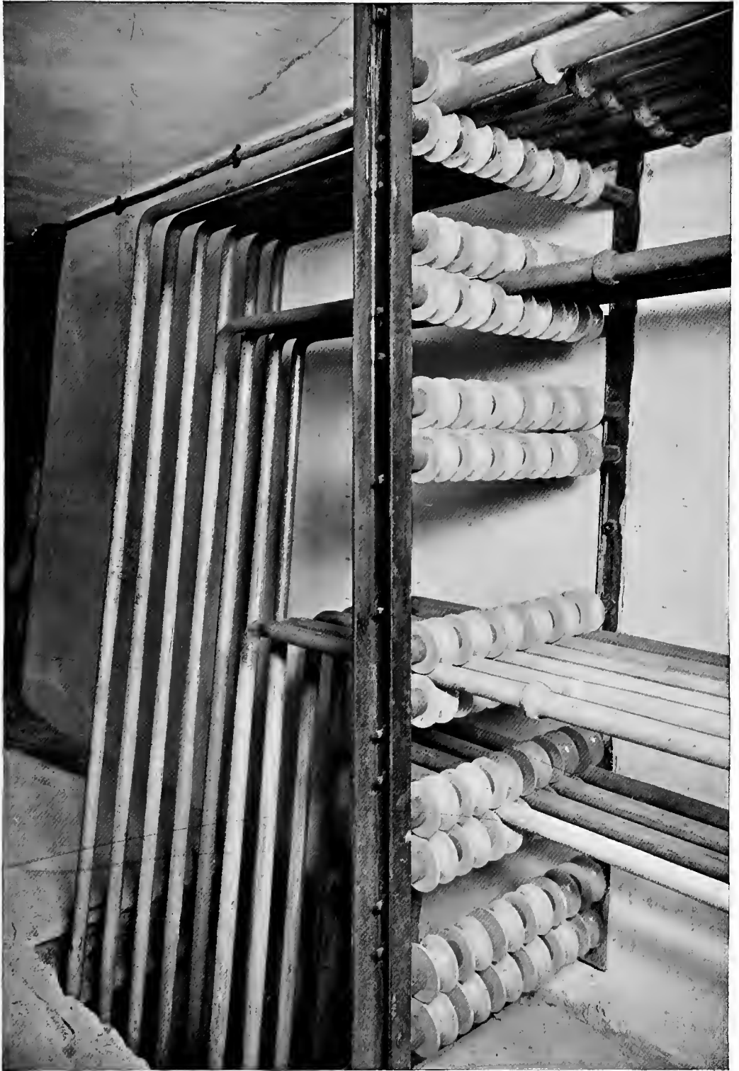
ALUMINIUM FEEDER CONNECTIONS BUTT-WELDED ON SITE (By courtesy of the British Aluminium Company, Ltd.)
